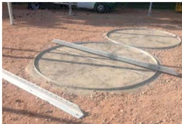
facilities is shown above. A set comprises of 5 sockets (with nylon cap for when not in use) and 2 galvanised angle irons. The holes for attaching straps are every 100mm. The number of fixing points back and front can vary, however a greater number will add flexibility as athlete throwing frames do not come in standard shapes and sizes.
